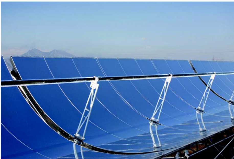
Figure 2. Parabolic trough concentrating solar collector.
