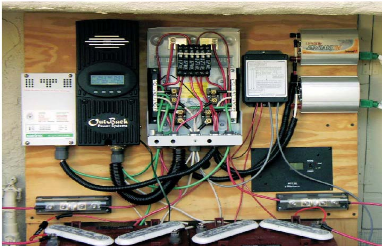
Figure 3. Power center for my dual PV system. Only half the parts are necessary for a more typical single system. Cut off at the bottom edge of the photo are two 12-V, 150-Ah batteries (one for each system), and immediately above them are 110-A class-T fuses. At left are two charge controllers. The black one is a maximum power-point tracking charge controller, as described in the text; it is certainly overkill for this small system. In the upper right are two 400-W inverters. Below them is an MPPT charge controller not currently used. To the left of the inverters is the monitoring system, capable of measuring two voltages and three currents. In the center is the exposed breaker box, showing three breakers per system, four shunts for current measurement (I use only three
