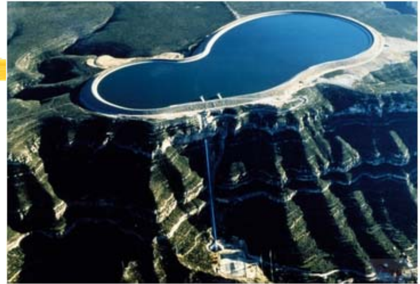
Pumped hydro in Spain: The upper reservoir of the Cortes-La Muela hydroelectric station in the municipality of Valencia, Europe's largest such facility.
